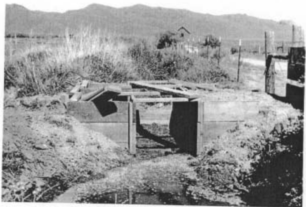
Diversion gate - Gillihan Ditch
